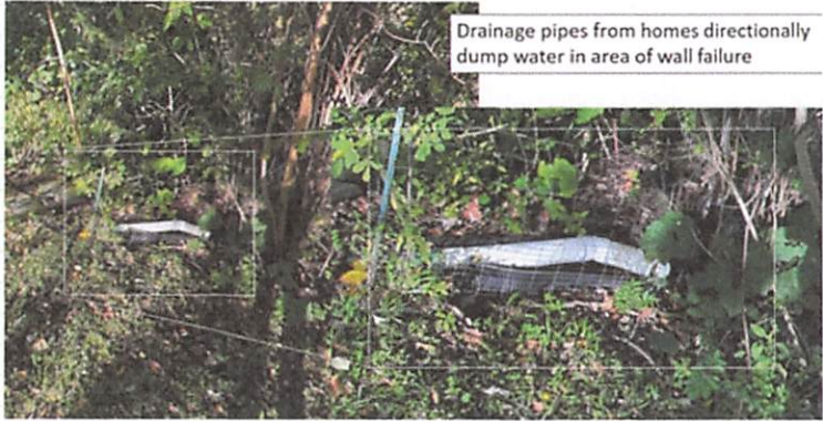
Example of Existing Drain line at the top of the Bayou Slope
